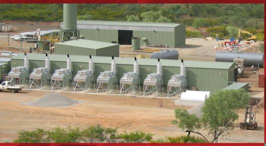
Contract Power launched **STAMFORD®** S9 to the fleet of eight **STAMFORD®** HVSI804R1 units for the 12 MW power plant at the Savannah Nickel Sulphide Mine, located in the East Kimberly Region of Western Australia. The Savannah Mine is one of the three mining projects in this region.
