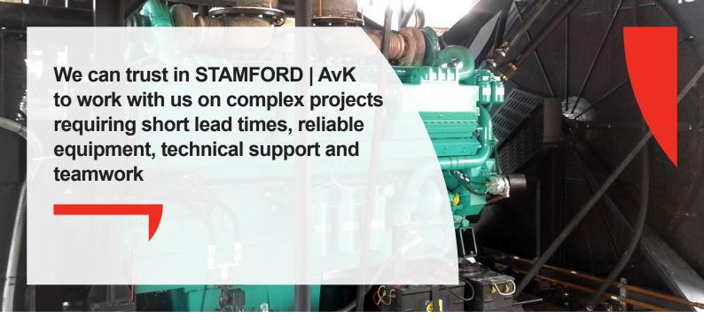
The complete system is an arrangement of four gensets that deliver 9MW of continuous power to a crude oil extraction site.
